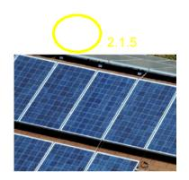
Underperformance of module 2.1.5 was automatically alerted by the system, and the module was remounted to avoid the shading as shown in the power curves
