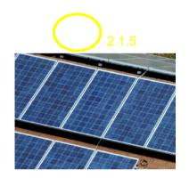
Module 2.1.5 (red curve) is partially shaded by the bottom right corner of the opposite module, as shown in the power curves
